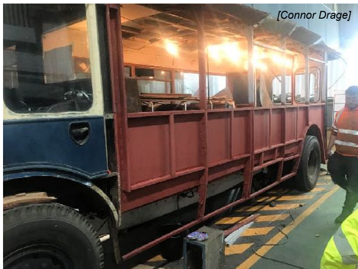
Notts & Derby 357's new framework and stress panelling.
